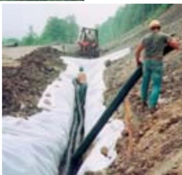
Left and inset: TerraTex SD Non-woven Geotextile (inset) from Hanes Geo Components aids in the filtration of water in highway edge drain applications, while TerraTex SD Woven Geotextile (left) separates native soil from pavement material to improve road stability and durability.
